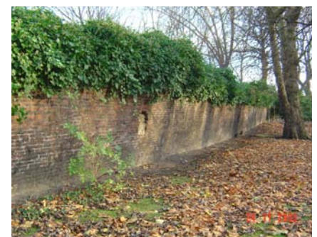
Fig.34 West boundary wall
