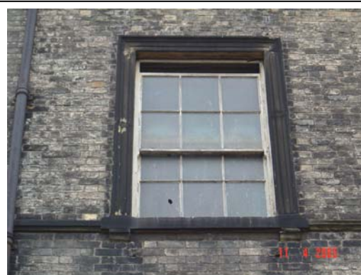
Fig.32 6-over-6 timber sash window
