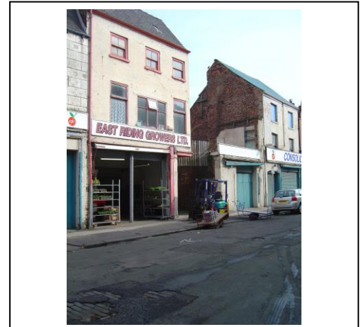
Fig.70 Concreted former town houses
