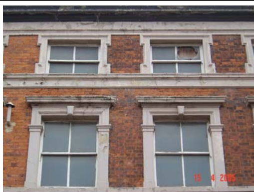
Fig.29 2-over-2 timber sash windows
