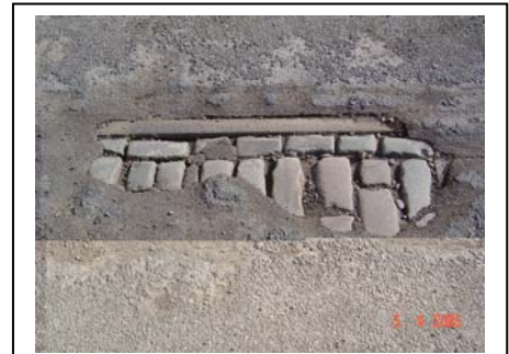
Fig.16 Concealed granite setts and railway line
