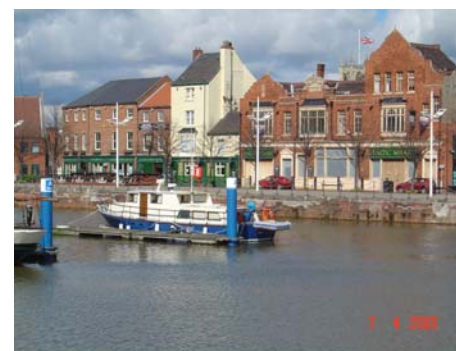
Fig.28 Traditional building & roofing materials
