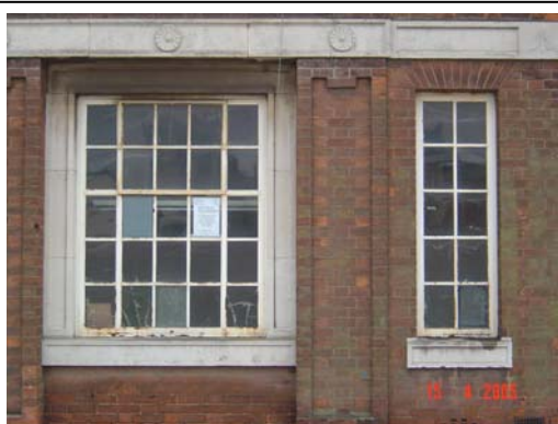
Fig.31 Metal casement windows
